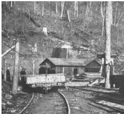
View of the mouth of a coal mine and surroundings after a fire. From U.S. Department of Commerce Bureau of Mines Bulletin 229: Fifty-nine Coal-Mine Fires: How They Were Fought and What They Teach by G. S. Rice, J. W. Paul, and M. W. von Bernerwitz (Washington, D.C.: U.S. Government Printing Office, 1927). From TRAIL collections.
